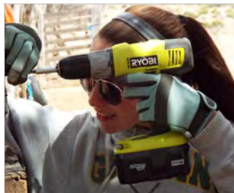
A Bishop Guertin volunteer installs a new gate at Ella's corral.
