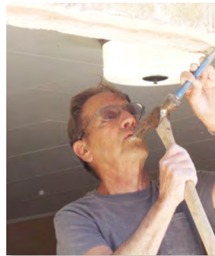
Bro. Robert prepares an opening for framing.
