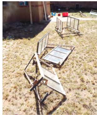
The original 1950s era windows didn't want to come out.
